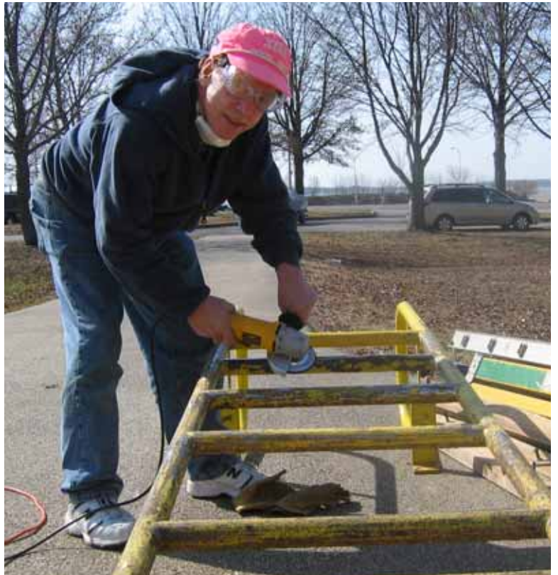
Don Crohn grinding rust and old paint from sea wall ladder
